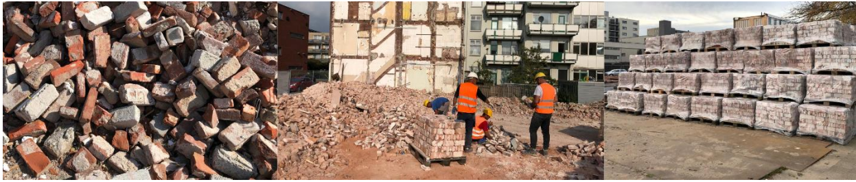
Figure 18. Brick Mining process, Rebrick, 2025
